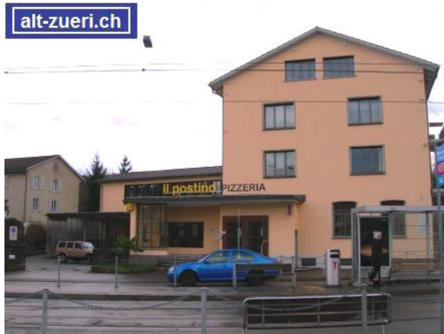
Rest. "Il Postino", Schaffhauserstr. 188, 8057 Zürich (Photo: Gebr. Dürst)
